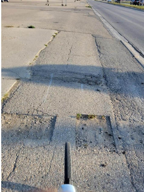
Photo: Hwy 12 Path near Loewen: Rough riding beside heavy traffic. In wet weather it becomes a 250m long "splash park".
